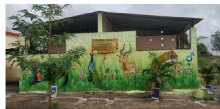
Project: Constructed 8 urinals & 2 WCs in each of 4 Zilla Parishad Schools.
