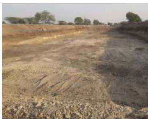
Work Site at Vadgaon-Gupta
