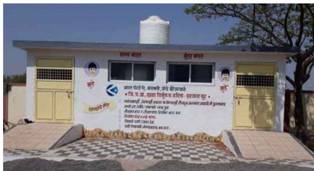
Project: Toilet construction Village: Shirsuphal Tal.: Baramati Dist.: Pune
