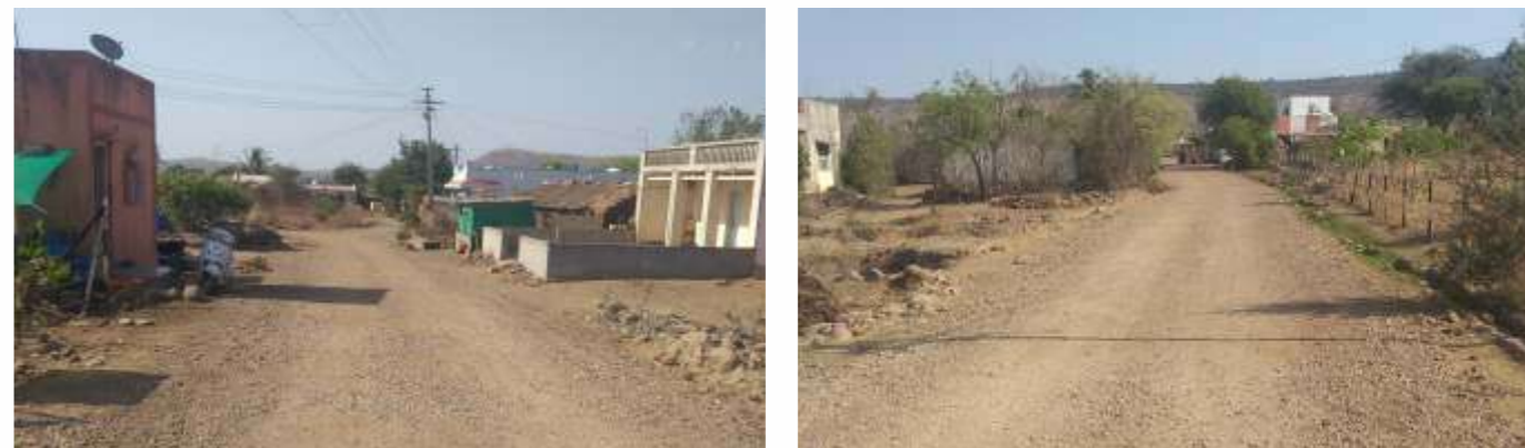
WBM Road at Nagzari
