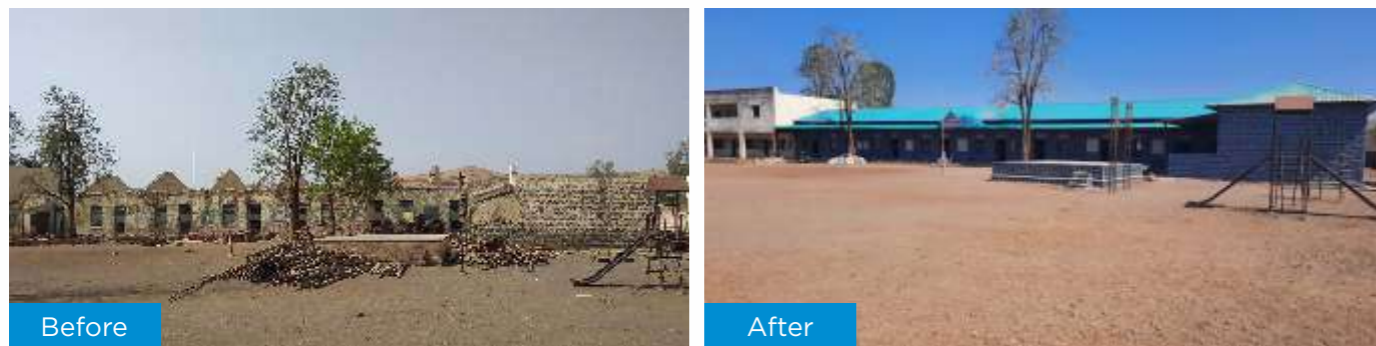
Project: Roof-work of Zilla Parishad School Village: Hivare, Tal.: Purandar , Dist.: Pune
