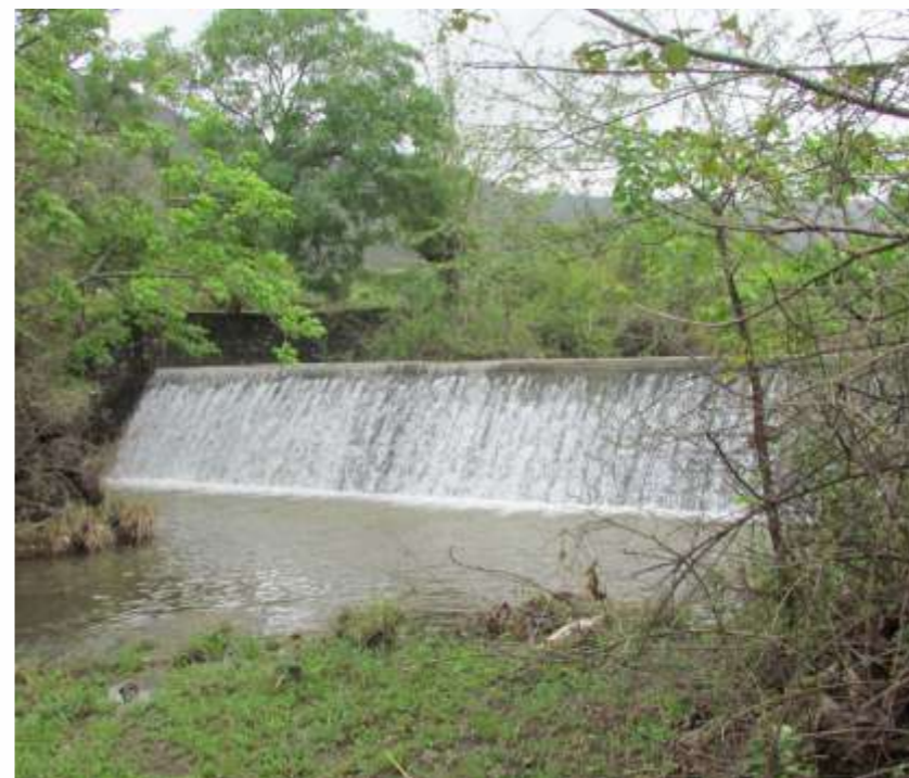
Desilting of cement nala bandhara work at Chapatewadi
