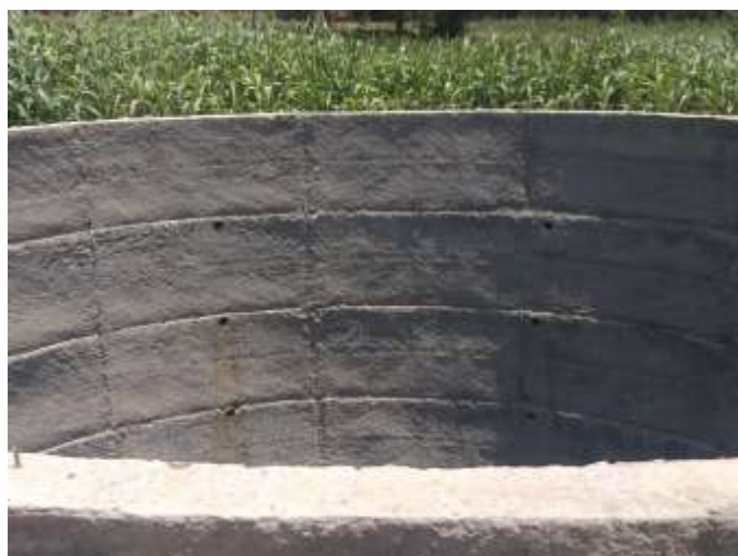
Construction of open well: Work completed & well was recharged after rains at Thakarwadi
