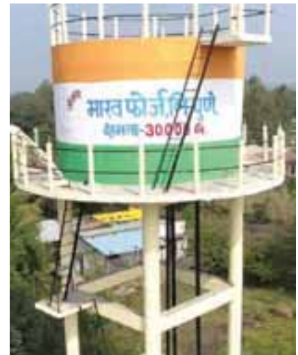
Constructed Drinking Water Tank District: Satara
