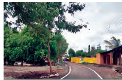
Construction of open gutters in Saygaon for Swachh Sunder Gaon competition
