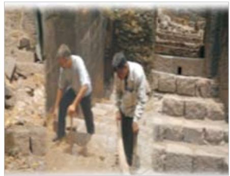
Repaired the steps at fort Purandar
