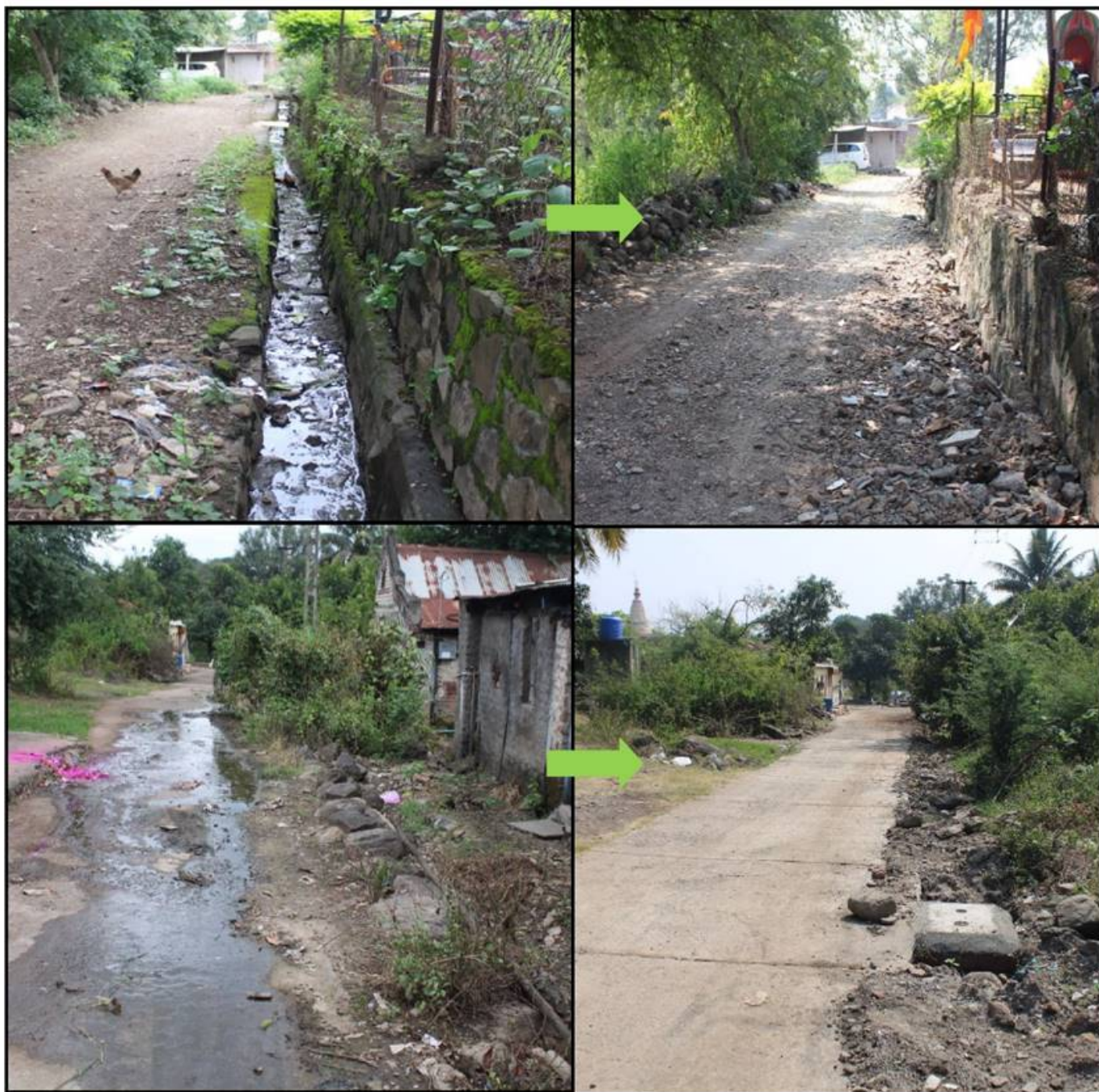
Construction of underground gutters at Apshinge
