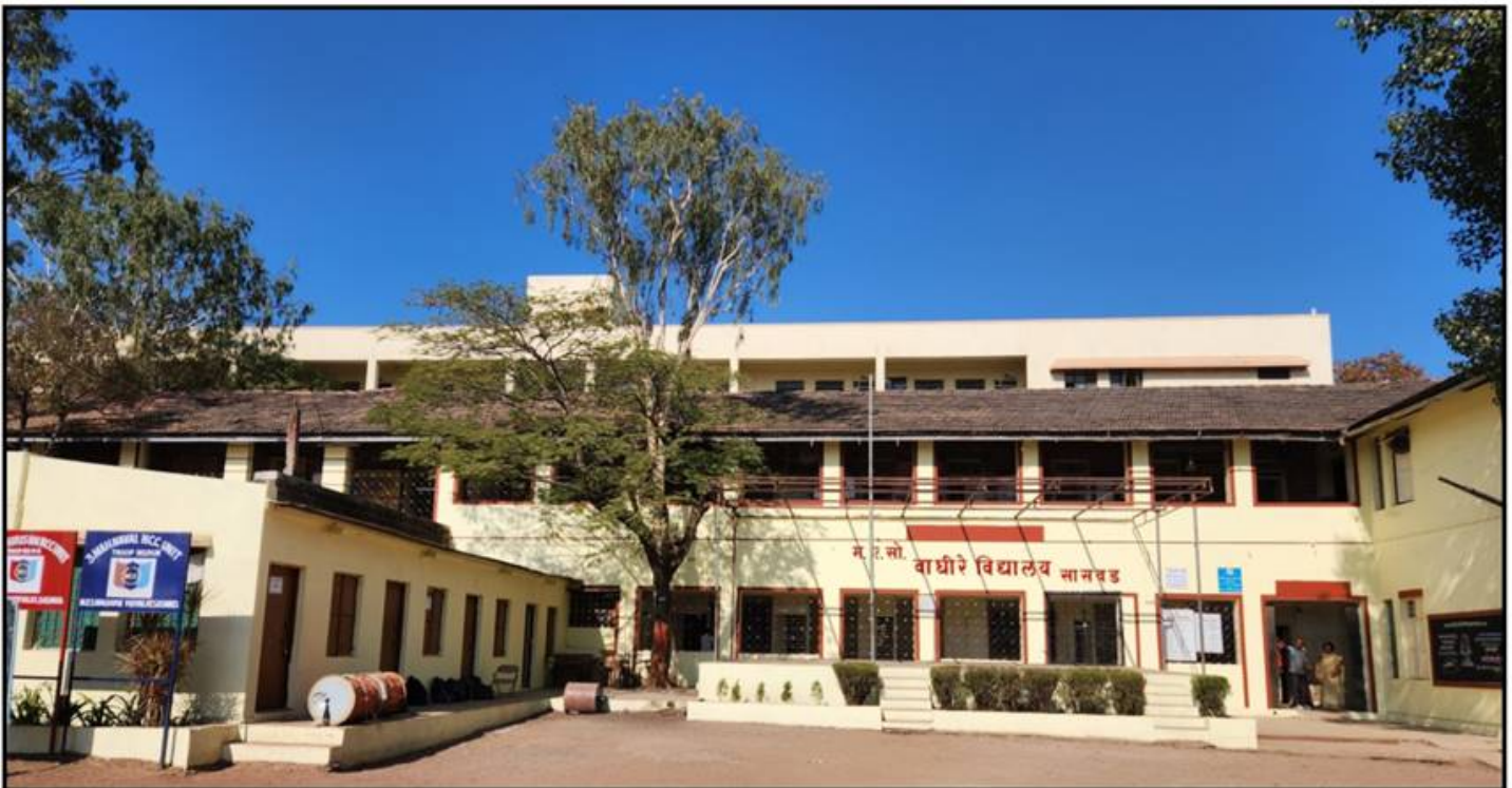
School building painting work at Saswad
