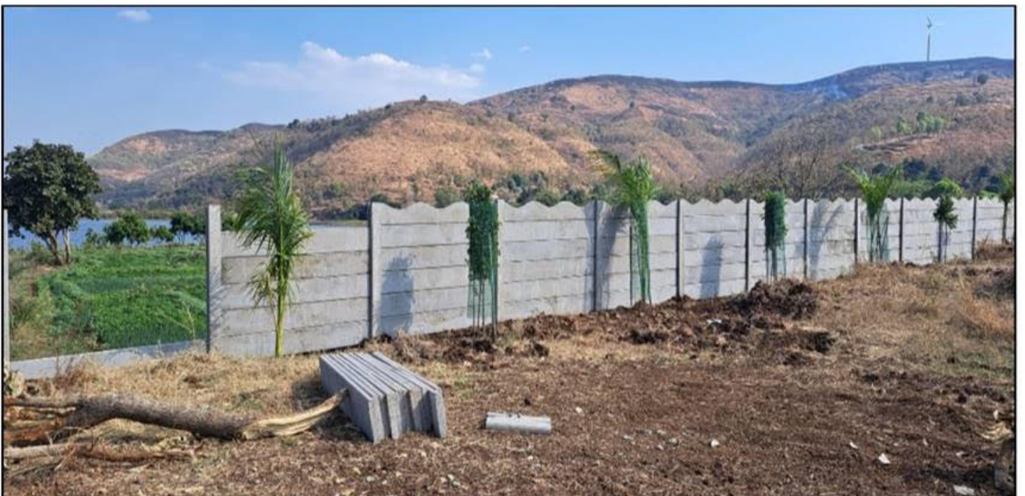
Construction of precast compound wall at village Salave
