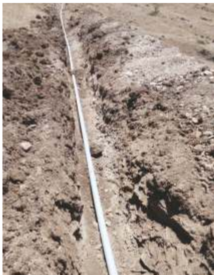
Pipeline laid for drinking water
