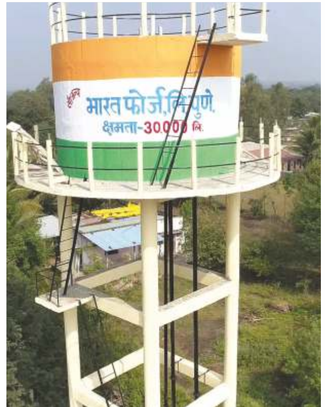
Drinking water tank construction
