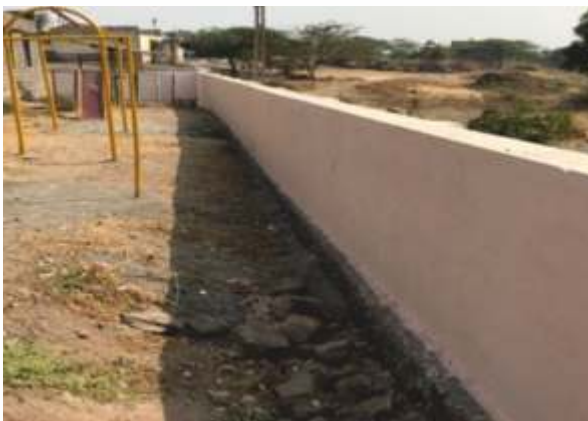
Compound wall construction
