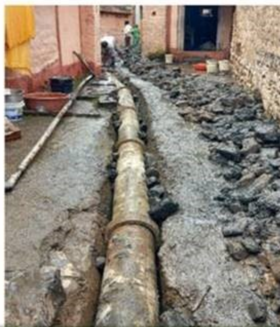
Construction of internal gutter at Jaygaon
