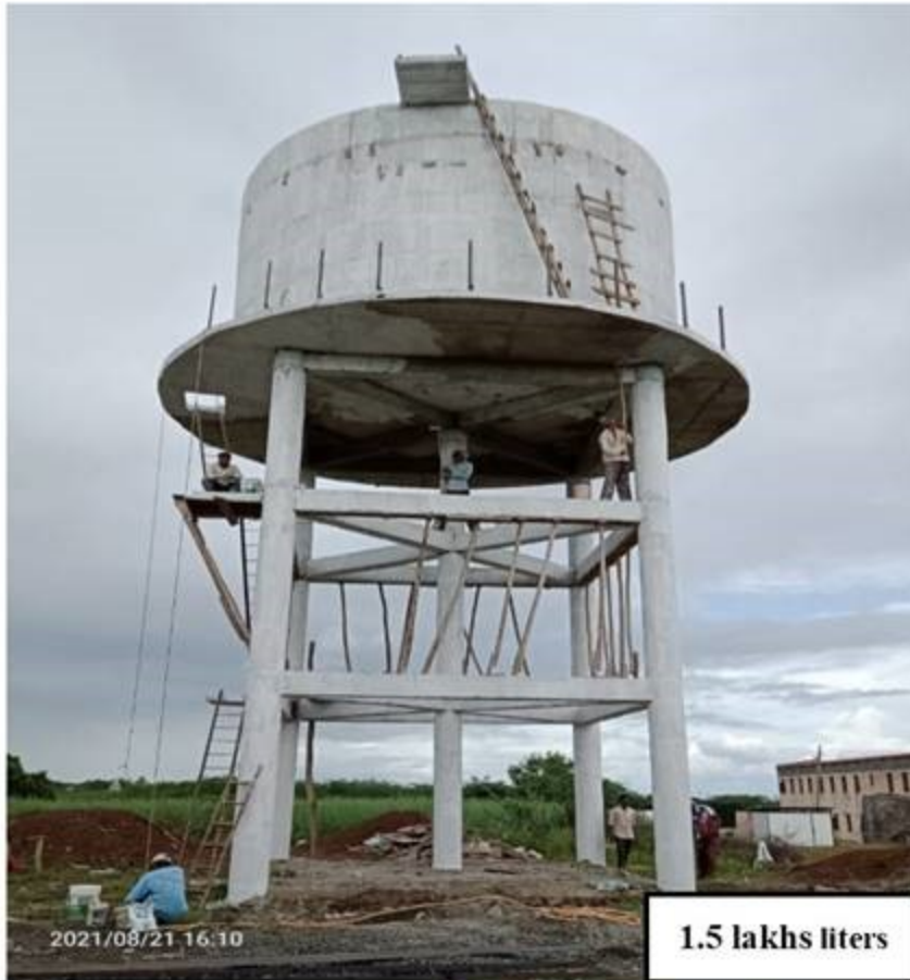
Construction of drinking water tanks at Gondawale
