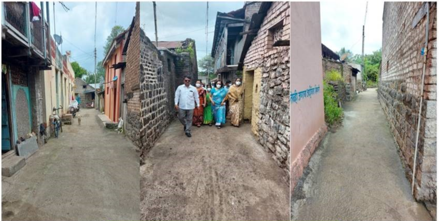
Construction of Internal roads and gutters at village Takale
