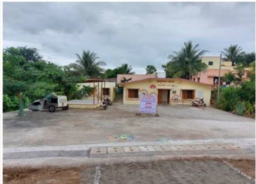
Room maintenance & floor work at Pimpari
