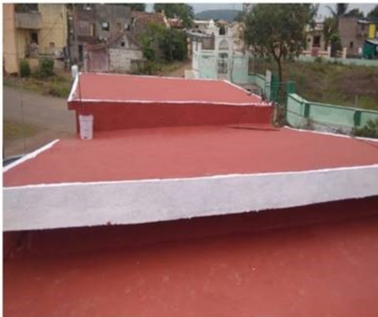
Water proofing work of the roof at Kalambi
