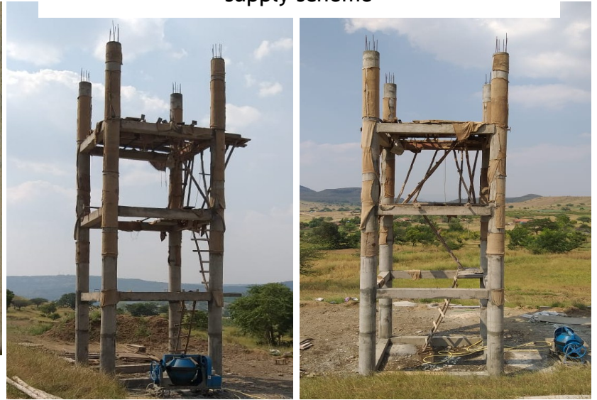
Construction of Water Tanks under water supply scheme
