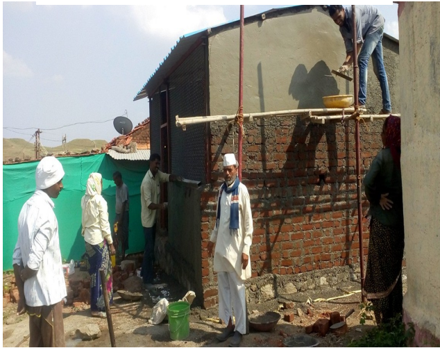
Construction of Cattle Sheds
