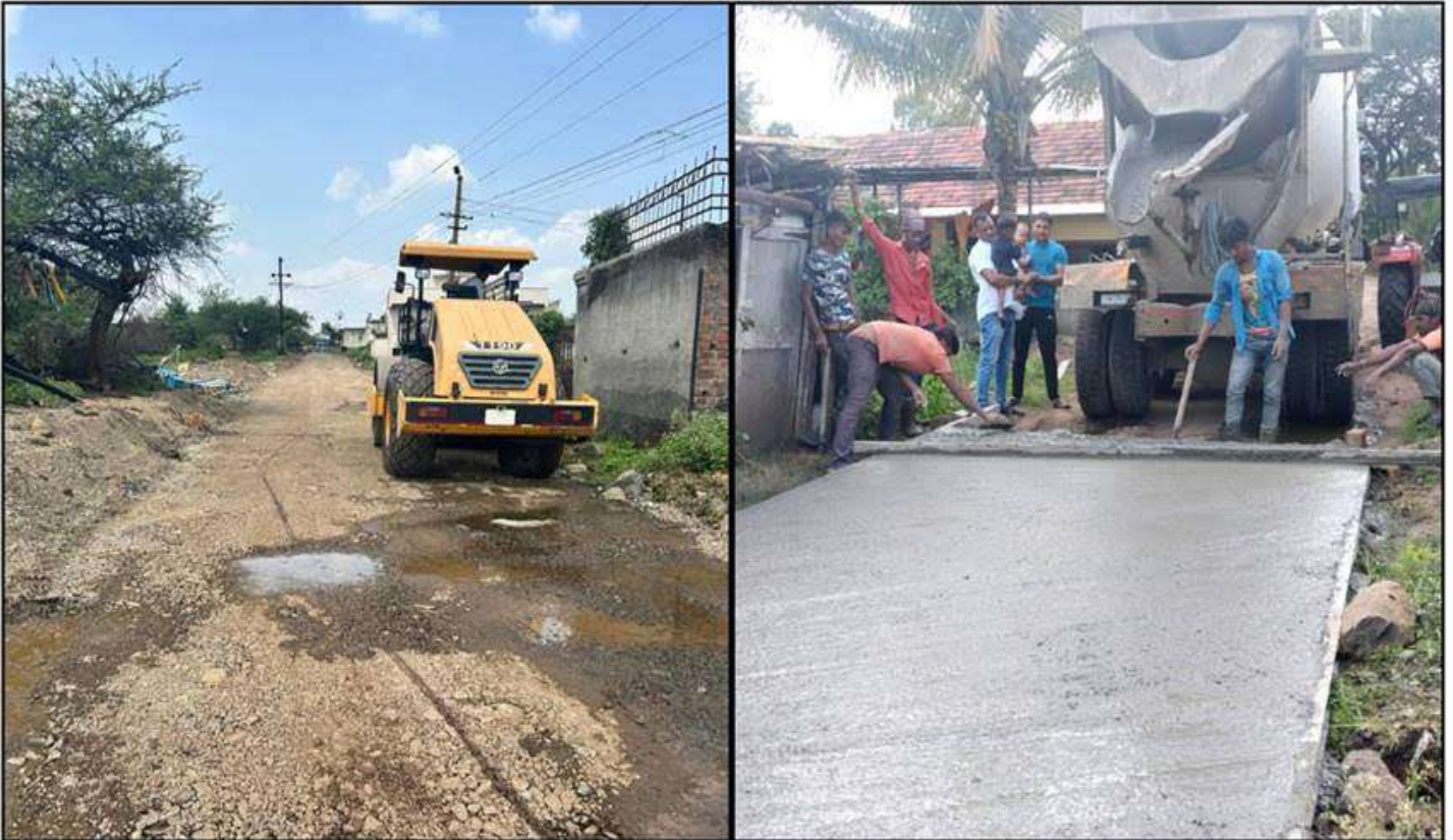
Construction of internal concrete & paver road at Bopgaon ,Bhivari & Hivare
